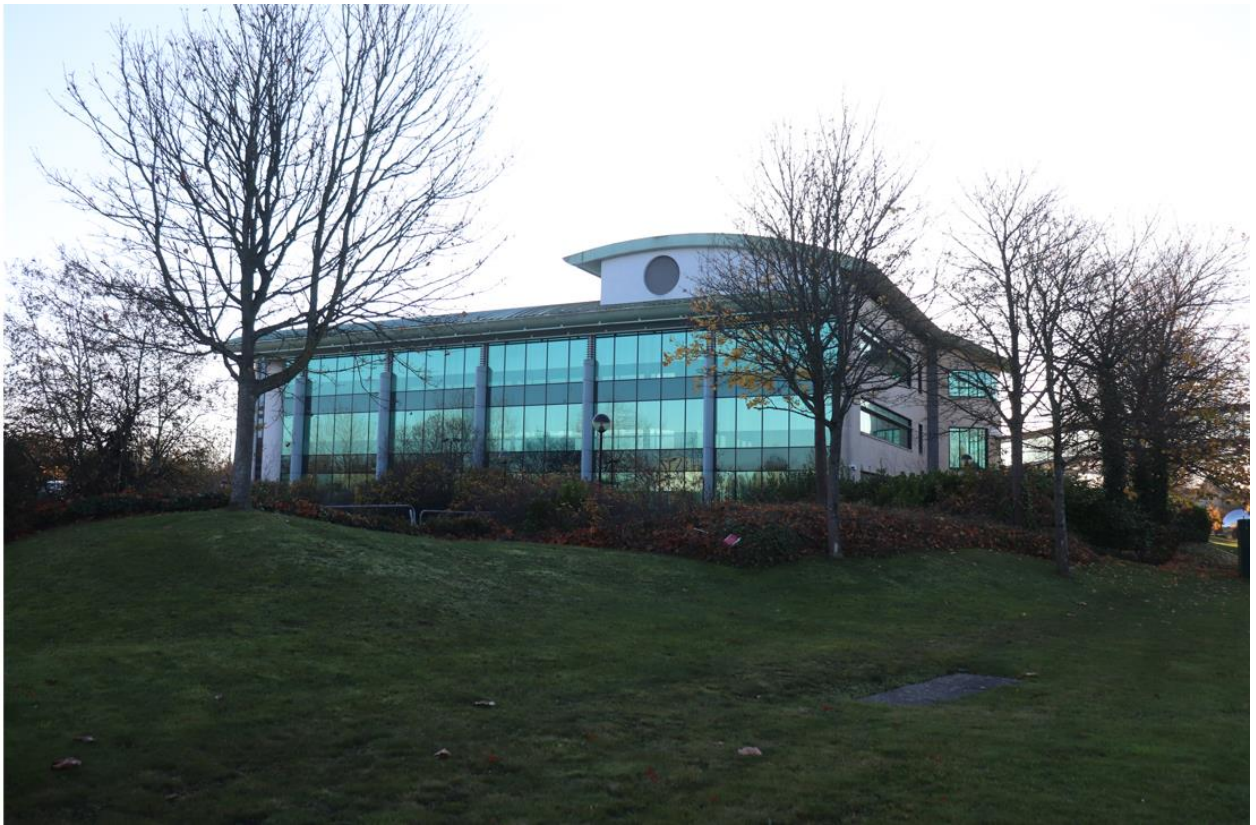
Application site from M3 Junction 3 (Building 1)
