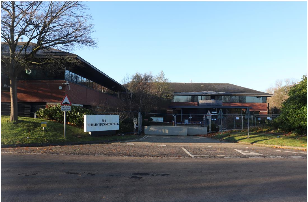
View from access road (Building 2)
